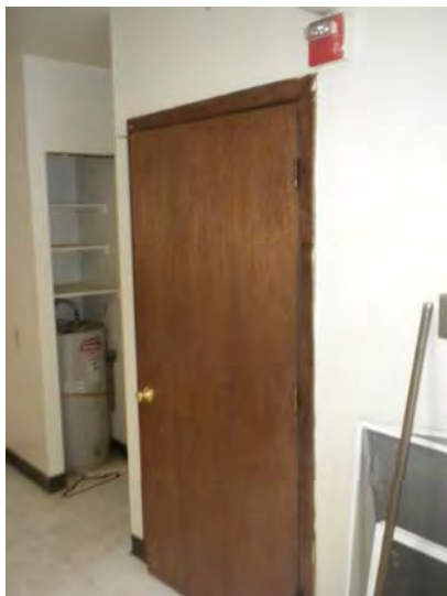
Interior closet door and horn/strobe on the wall
