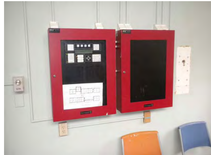
The central fire alarm control panel
