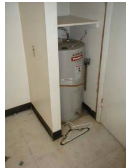
View of an electric domestic hot water tank
