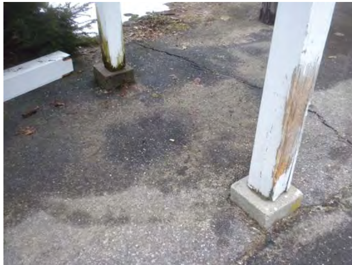
Example of wood rot and damage to the wood posts supporting the walkway canopy
